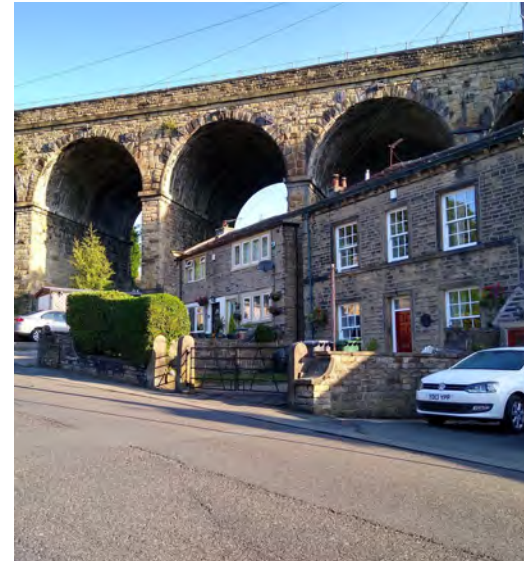
A railway viaduct meeting domestic character in Slaithwaite.
