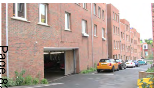
Undercroft and on-street parking provided at the Malings, Newcastle to ensure the development maximises development density
