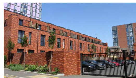
An internal courtyard provides car parking at Carpino Place, Salford to allow the front of the buildings to interact with the street
