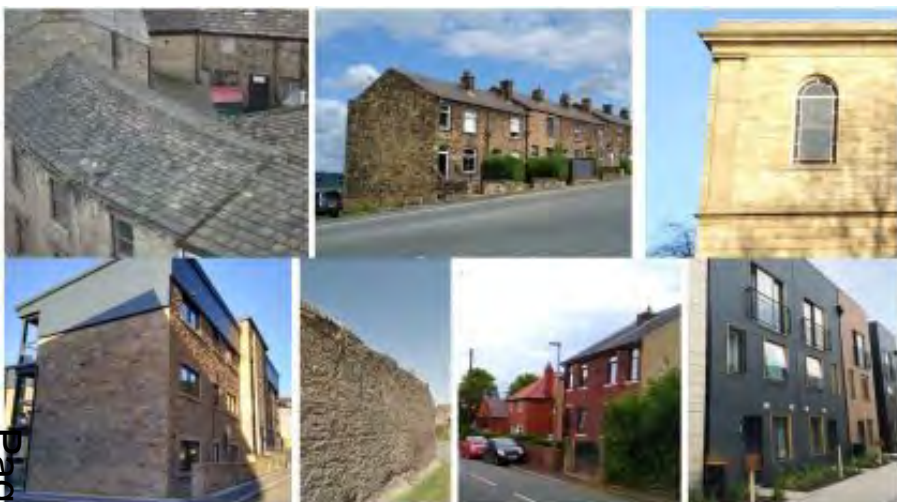
Clockwise from top left: stone roofs commonly found in Kirklees, stone terrace with slate roof at Thornhill, ashlar stone in Dewsbury, contemporary modular housing (Image:Citu), red brick housing at Whitley Lower, coursed rubble at Denby Dale and contemporary stone buildings at Slaithwaite.
