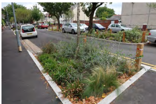
Natural solutions to drainage, which also provide visual amenity in the streetscene at Greener Grangetown, Cardiff (Image: Susdrain, Flickr)
