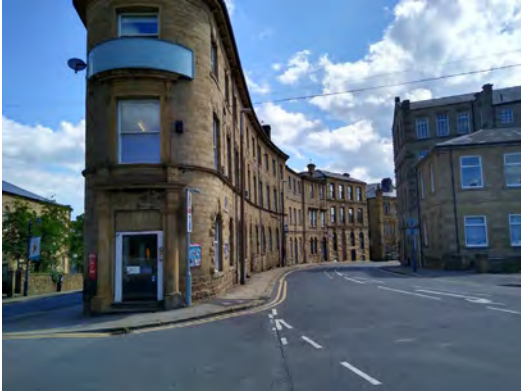
Former textile warehouses creating a high quality urban townscape in Dewsbury Town Centre
