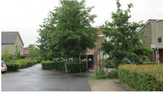
A well screened communal bin store at Staiths South Bank, Gateshead
